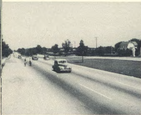
The southbound lane of Du Pont Parkway. This is U. S. Highway 13 and 40.
