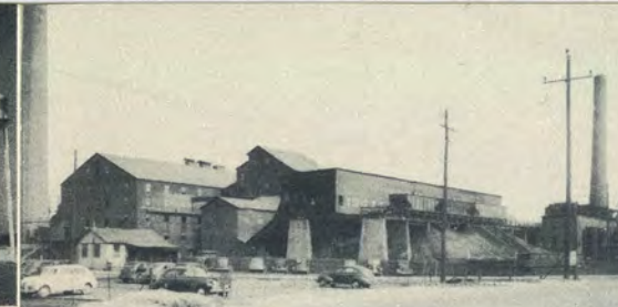
The Pyrites Company. This plant extracts copper from pyrites iron and cinders the residue into iron ore.
