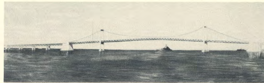
The Delaware Memorial Bridge.
