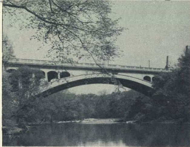
The City of Wilmington obtains its water supply from the beautiful and historic Brandywine River.
