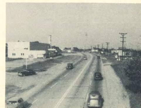
By-pass of U. S. Highway 13 north of Wilmington.
