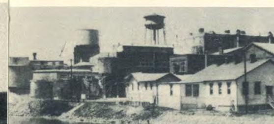
DuPont Company's plant pigment manufacturing unit at Newport.
