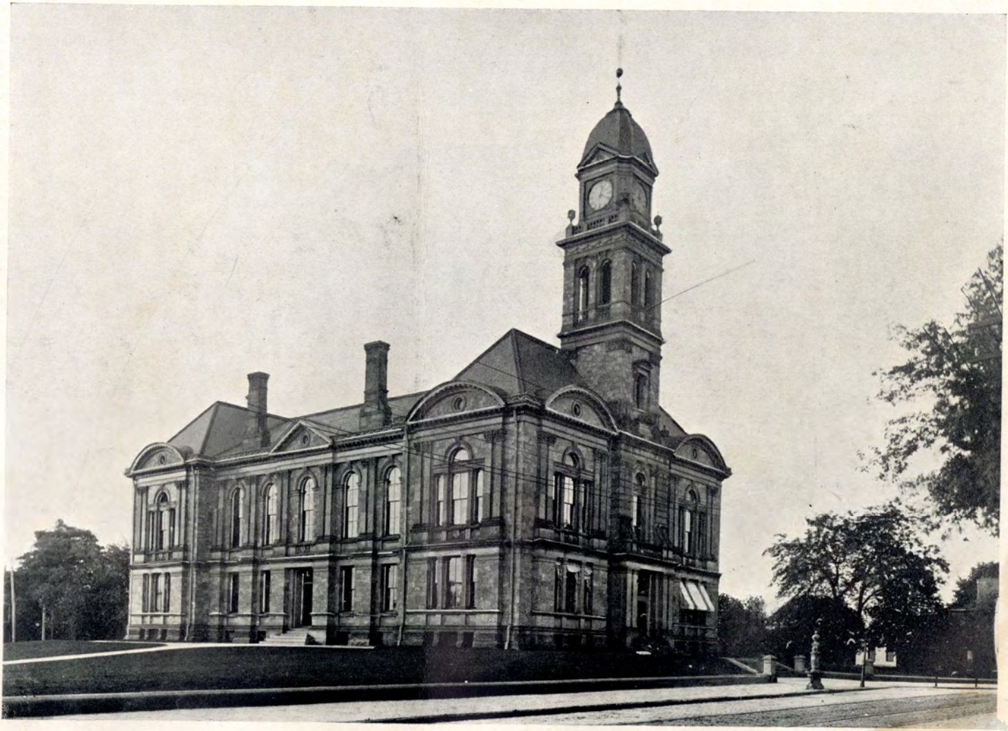
NEW CASTLE COUNTY COURTHOUSE
