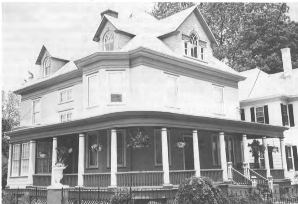
FIGURE 11: 105 WEST SIXTH STREET
