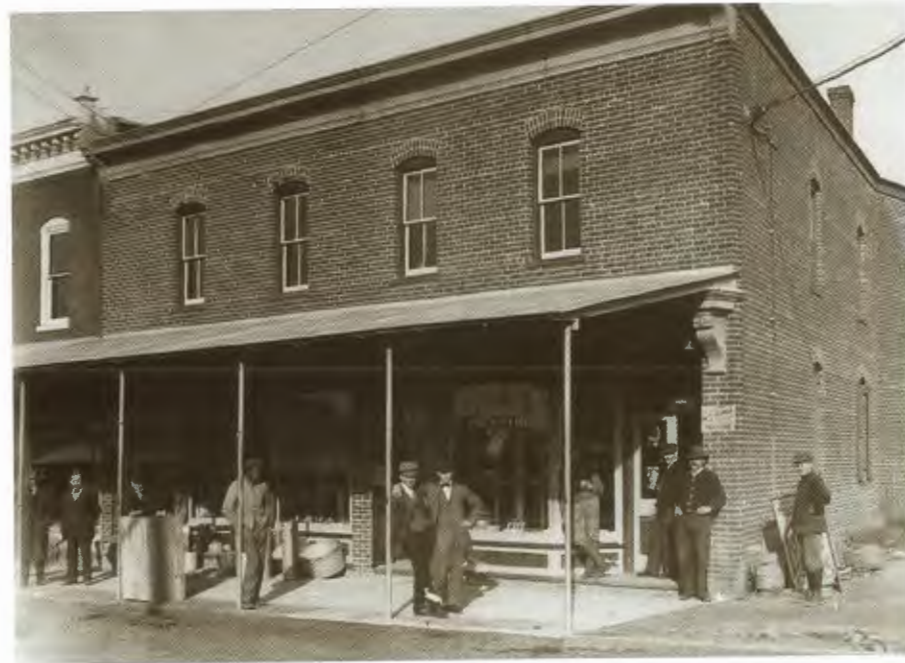
Another view of Union Street stores with the store of C.A. Conner, and the Central Cigar and Tobacco shop on the right. (Courtesy of Donald Carey)
