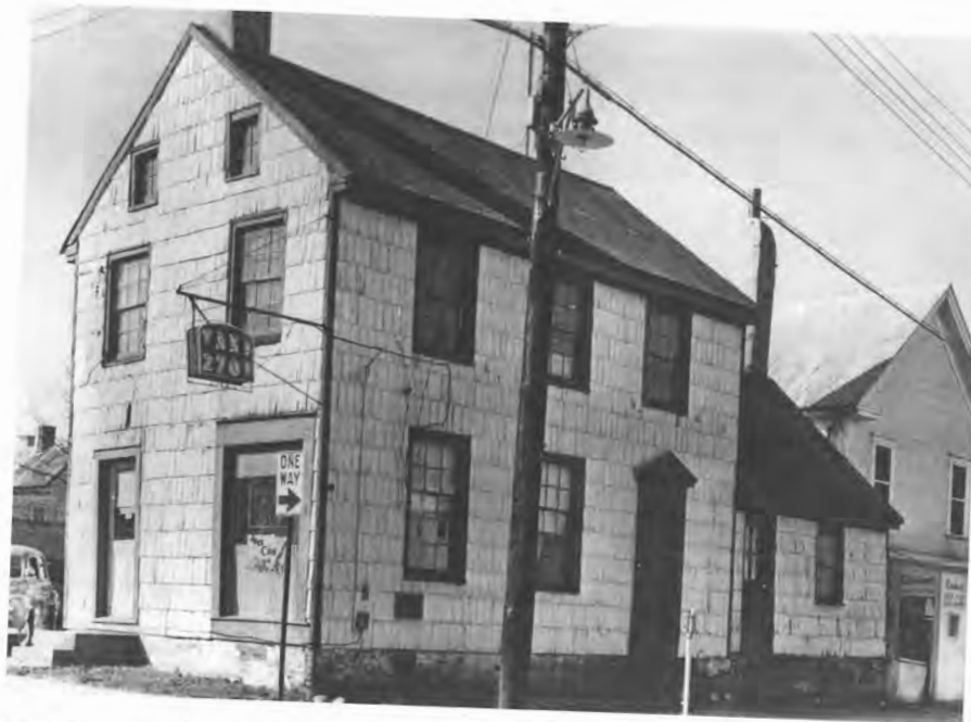
The Cannonball House before it was restored and turned into a museum. The cannonball is lodged in the large dark square in the foundation of the building. Courtesy of the Delaware Public Archives.
