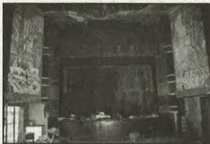
The Milton Theatre is shown before renovations.
