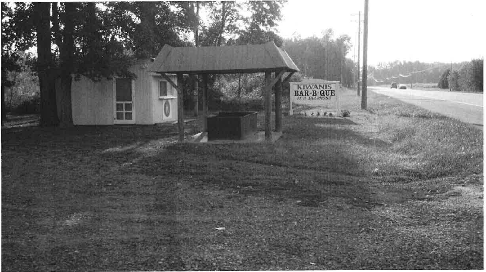
DE_Sussex County_Hebron M.P. Church view of adjoining property west of church 16 of 16
