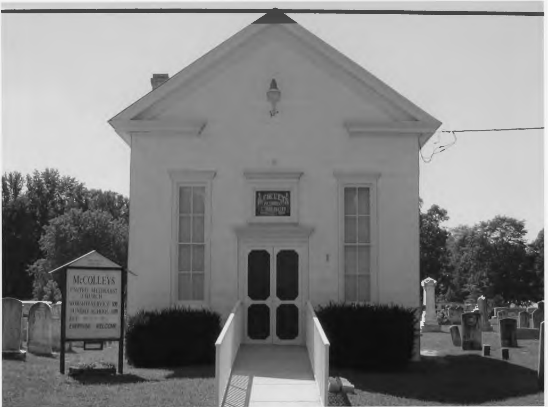
McColley's Chapel Sussex County, Delaware Facade View
