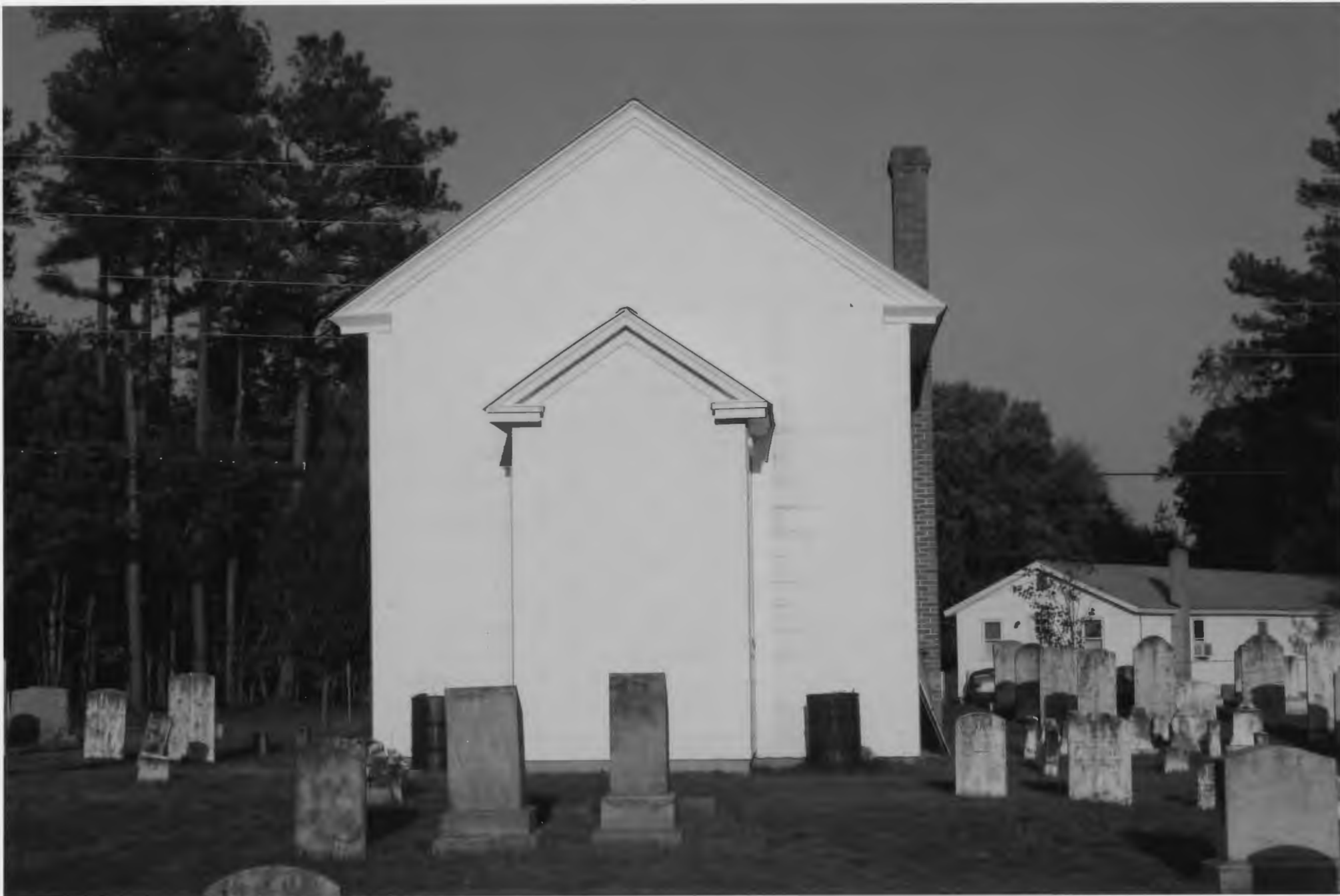
Mc Colley's Chapel Sussex County, Delaware rear elevation
