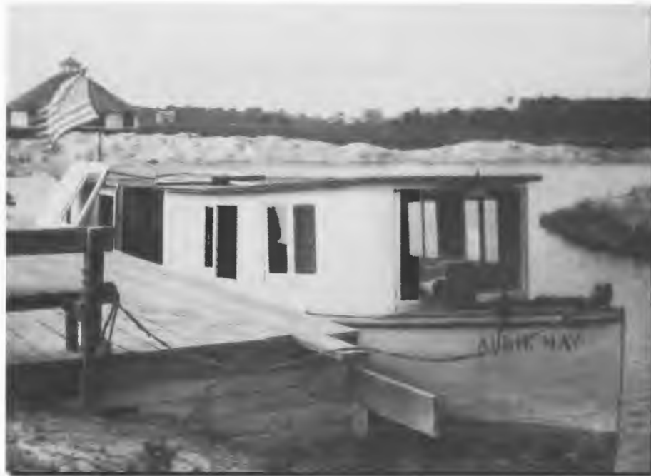
After the loop canal was built, passengers traveled on the Allie May to their final destination. John Addy's son Will was in charge of the loop canal construction, which was completed on July 8, 1910. The tabernacle is visible behind the flag.
