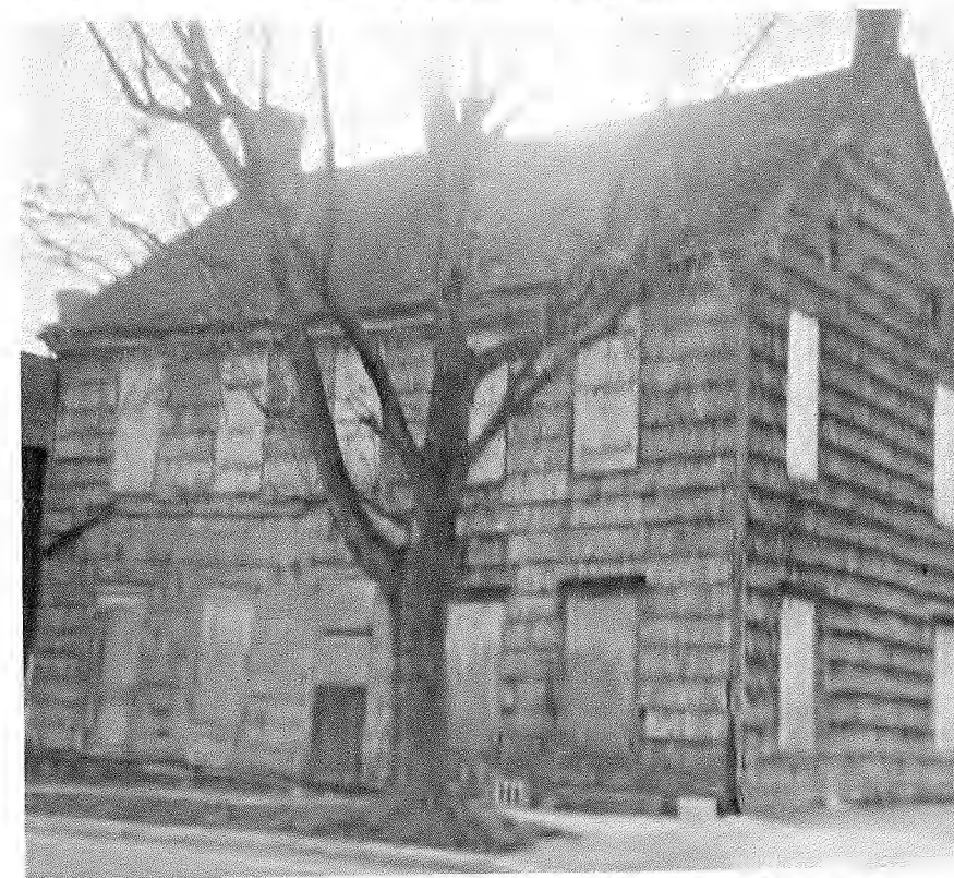
Georgetown's original courthouse on its South Bedford Street site prior to restoration.
