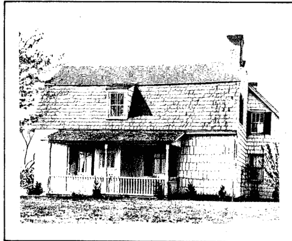
Maull House in 1937 before restoration
