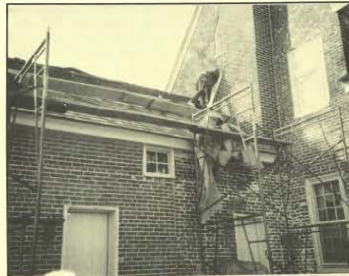
Restoration in progress on rear of Mansion.
