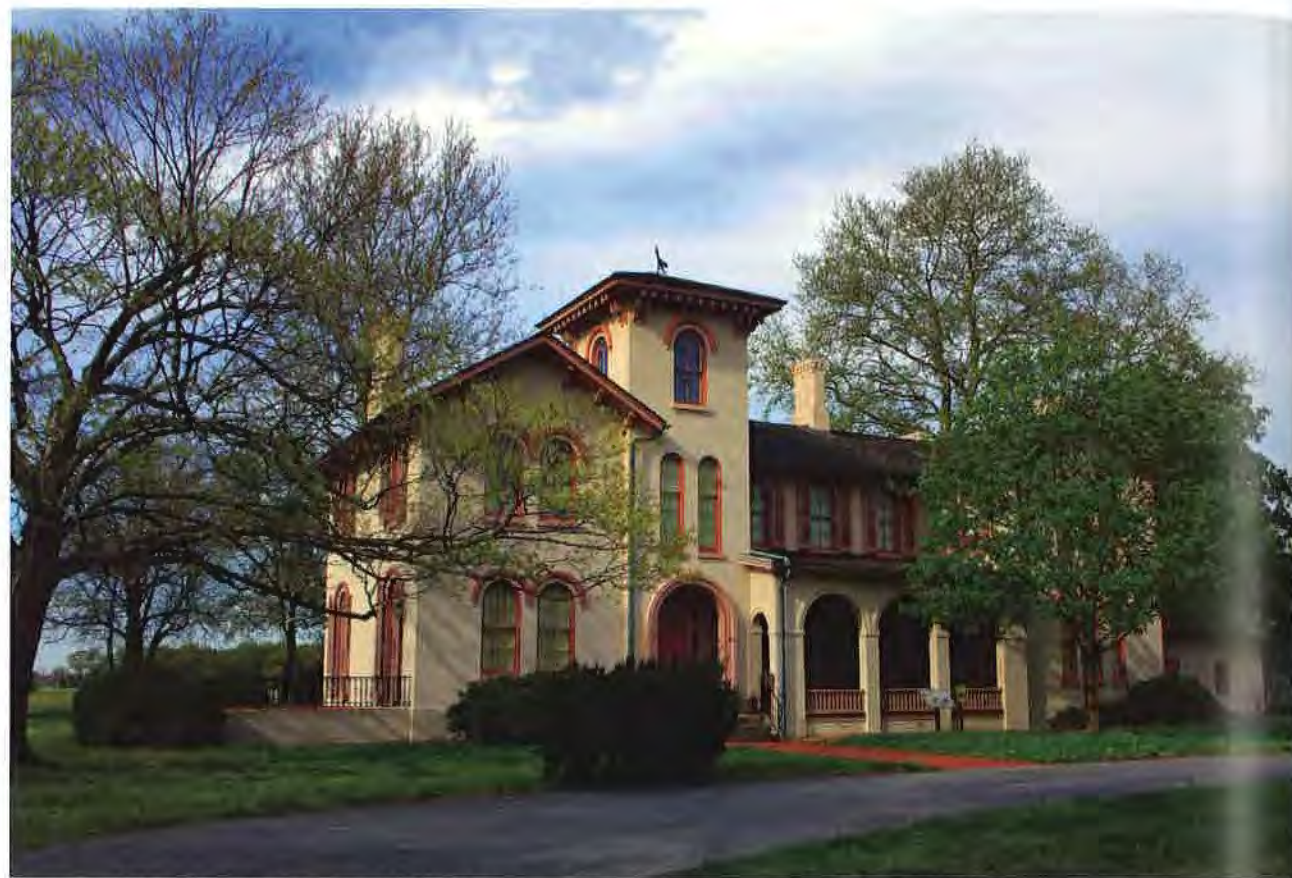
The Ross Mansion, built between 1854 and 1860 on the extensive plantation of former Governor William Henry Harrison Ross north of Seaford. The structure, now maintained as an historic site by the Seaford Historical Society, is one of the finest examples of Italianate architecture in the State of Delaware and one of Sussex County's most beloved historic landmarks (photo by Dick Carter).
