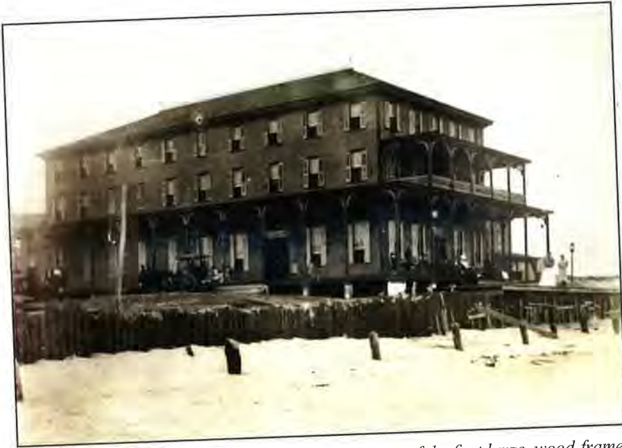
The Bright House hotel at Rehoboth Beach was one of the first large, wood-frame hotels of the resort's early days.
