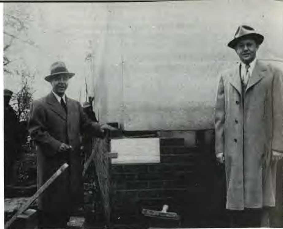
Mr. Stone, left, is shown in late 1950 at ceremonies marking the laying of the corner stone of the new educational building. At right is W. Allen Hastings, contractor and member of the congregation. The new unit includes educational facilities, a well-equipped kitchen, and a large social room. It affords space for eight classrooms and a lounge on the first floor.
