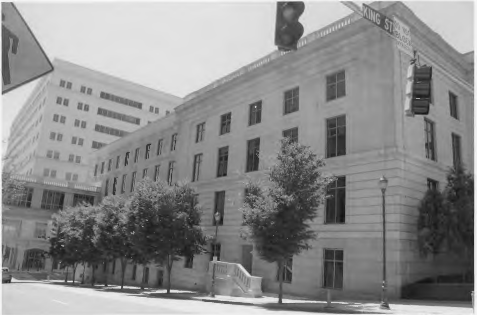
Rodney Square Historic District - New Castle, DE Wilmington Public Building, North Elevation view southeast
