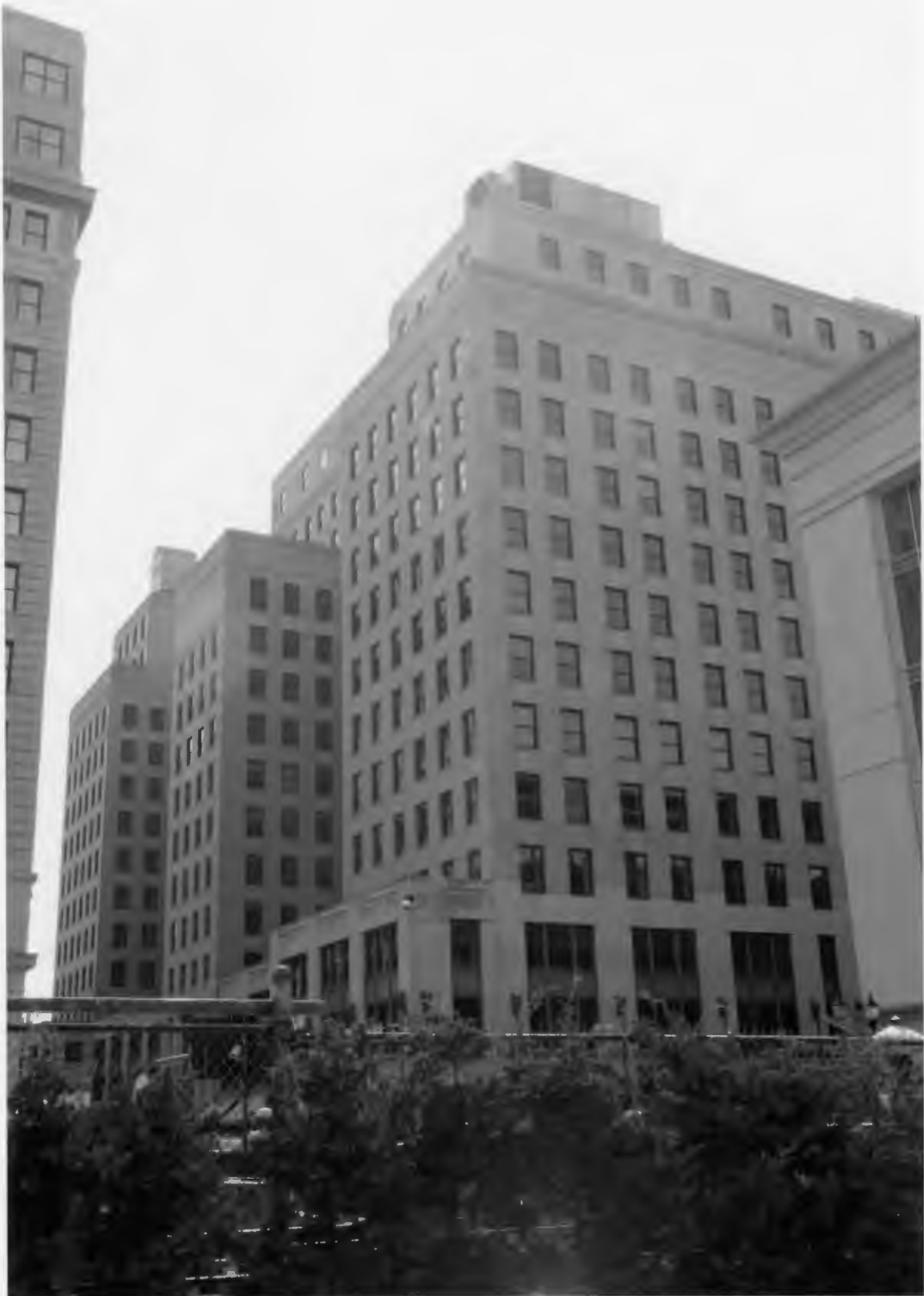
Rodney Square Historic District - New Castle, DE Nemours Building, North and East elevations, view southwest
