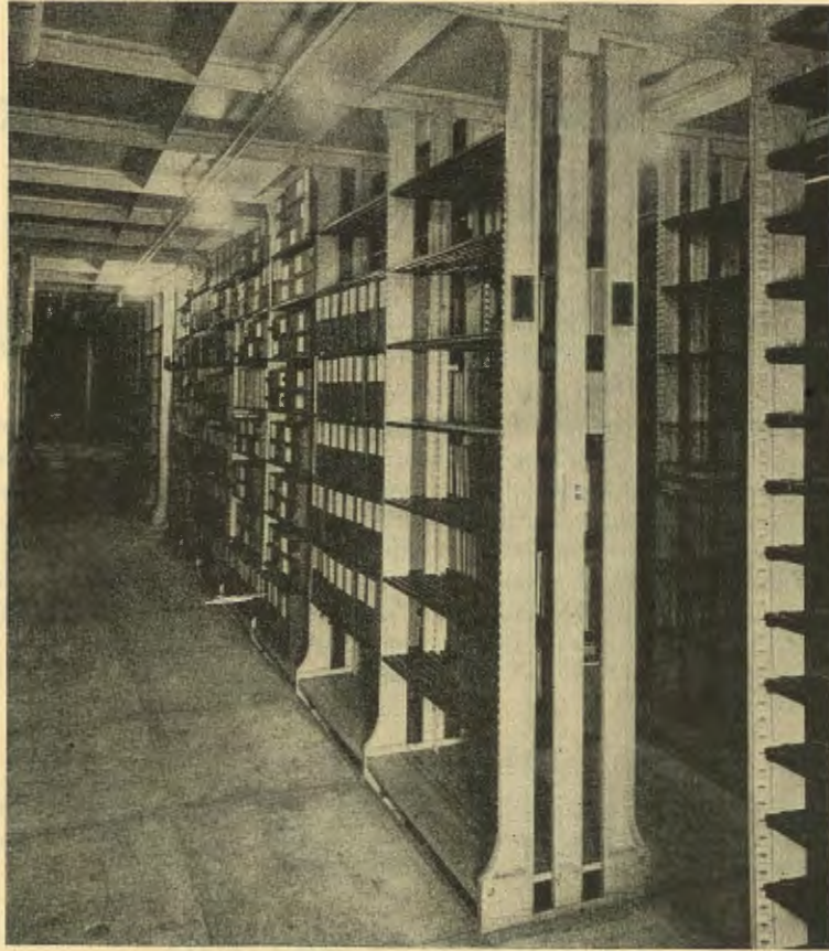
VIEW OF SNEAD STANDARD TYPE A STACK, WILMINGTON PUBLIC LIBRARY, WILMINGTON, DEL.
