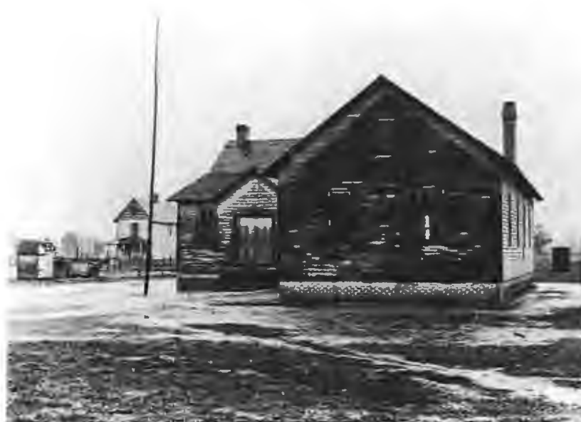
Bridgeville Colored School, Sussex County Courtesy of Hagley Museum and Library
