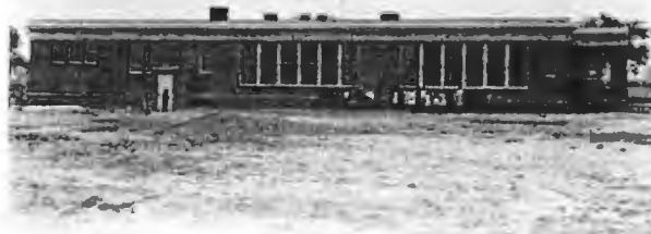
Bridgeville Colored School, Sussex County Courtesy of Hagley Museum and Library
