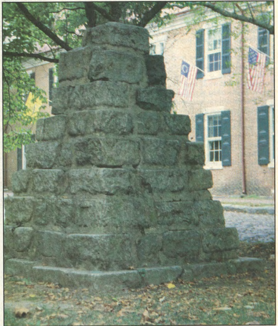
Wooden rails for the New Castle to Frenchtown Railroad were supported on stone supports known as "sleepers." These sleepers are on display as part of a monument in Old New Castle.
