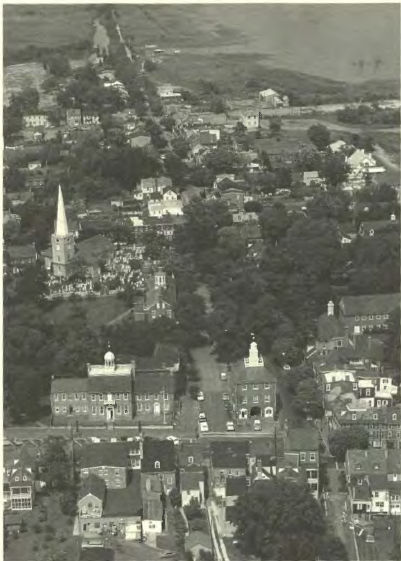
Detail from aerial view of New Castle, ca. early 1960s. (Courtesy of the Historical Society of Delaware.)
