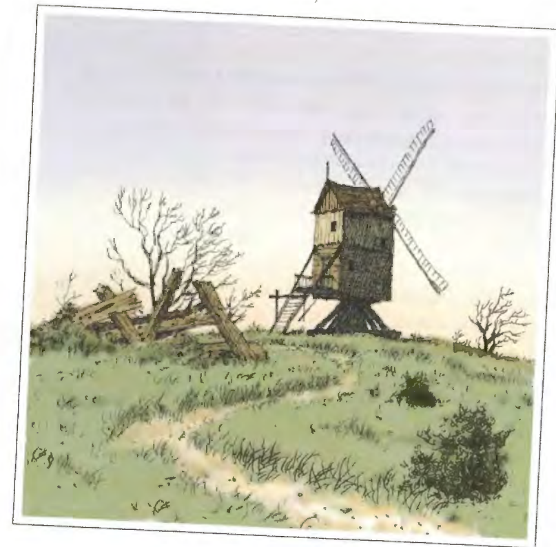
Arnoldus de la Grange built a windmill, circa 1681, on the inland side of the ruins of Fort Casimir.
