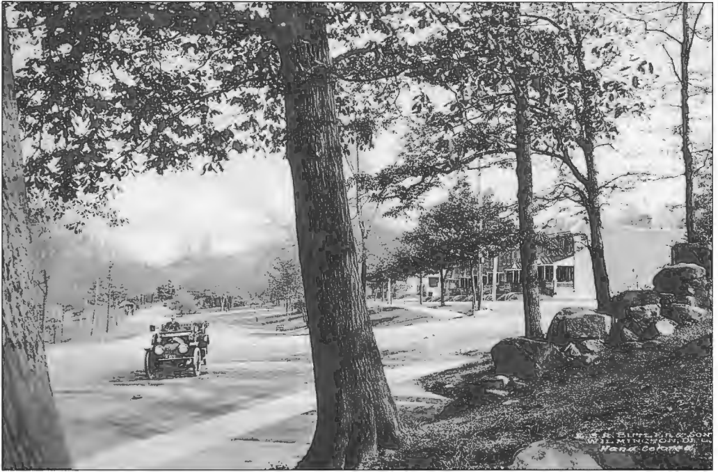
Brick row houses line Wawaset Street running parallel to Park Drive in Brandywine Park at Van Buren Street. The same location in the 21st century is nearly unchanged with the exception of a traffic light and the interstate overhead. This view of the park is around 1915. (Courtesy of the Hagley Museum and Library.)
