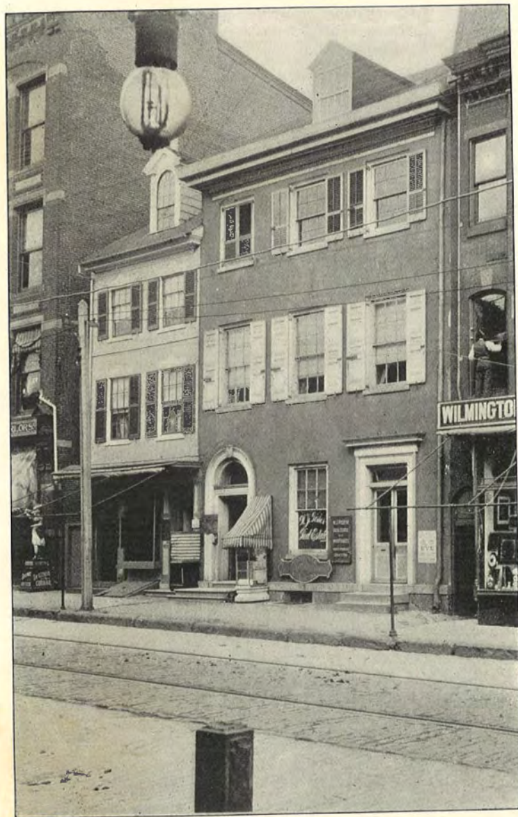
THE CITY RESIDENCE OF GUNNING BEDFORD, JUNIOR. NO. 606 MARKET STREET, WILMINGTON, DELAWARE.
