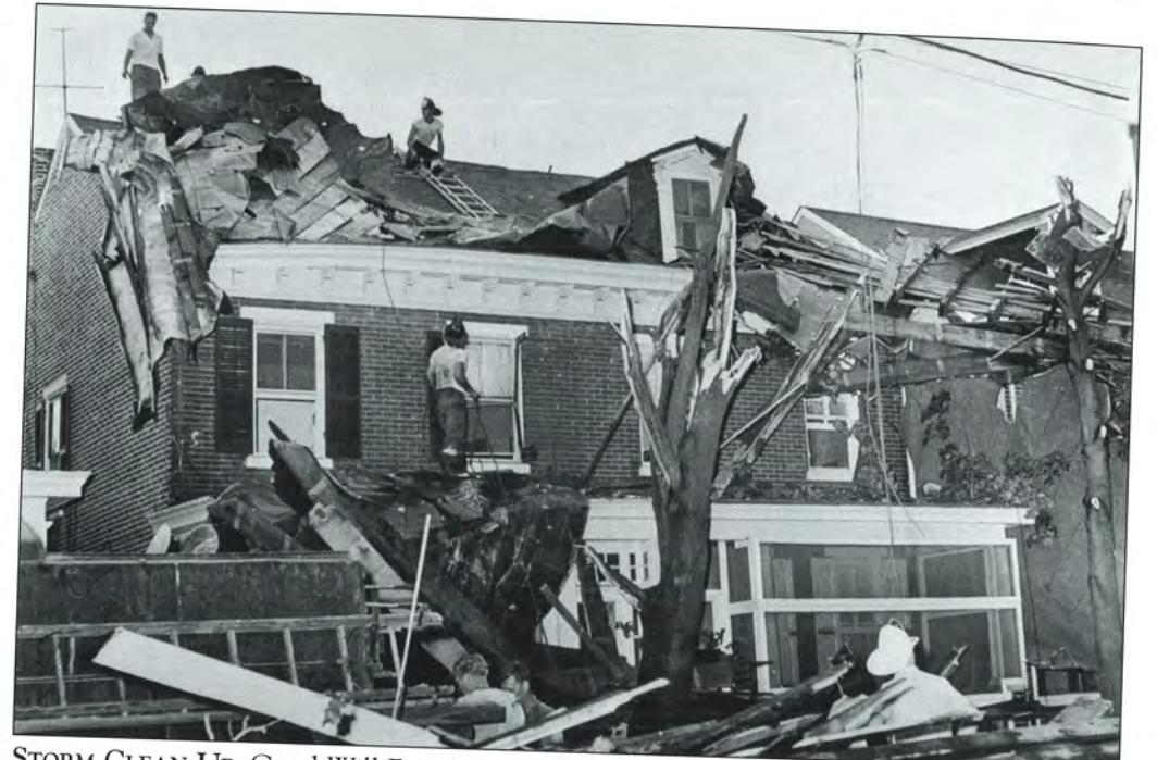
STORM CLEAN-UP. Good Will Fire Company members remove debris after the entire roof of Eliason Lumber Company's storage facility on South Street was lifted off and thrown about 40 feet north along Fifth Street in 1963. Due to the extensive damage from the violent storm, the building was demolished, but these homes were saved. (Courtesy of Ervin Thatcher.)
