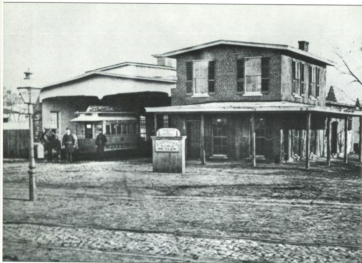
Heald and his partners began to set into motion plans for organizing the Wilmington City Railway Company (WCRC). The WCRC opened for operation with 7 horse-drawn trolley cars and 35 horses in 1864. This photograph of the car barn was taken September 8, 1883. The car barn site was nestled in the city block bordered by Delaware and Gilpin Avenues and Clayton and DuPont Streets. In the beginning, the car barn complex housed a car barn, waiting room, stables, and a blacksmith shop. (Courtesy of Hagley Museum and Library.)
