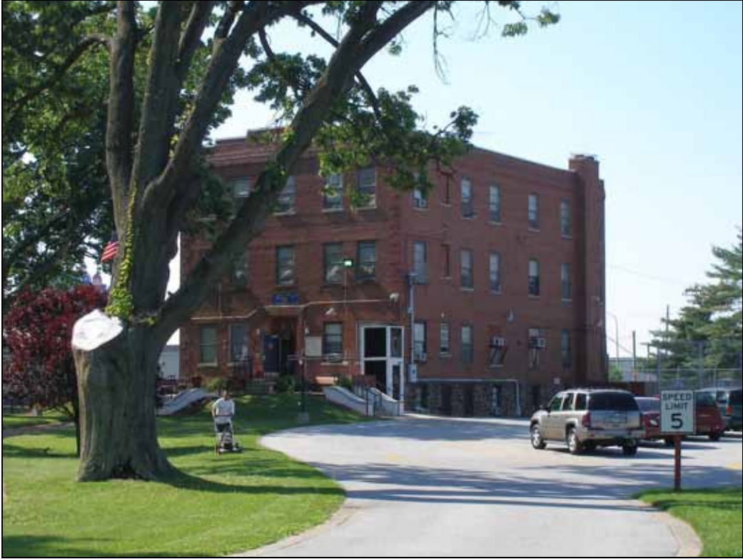
View of the facade and west elevations from the existing entry, looking southeast.
