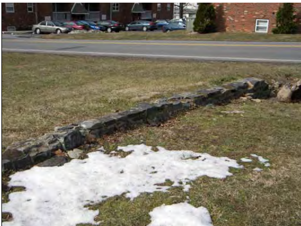
View of the stone wall looking southwest.
