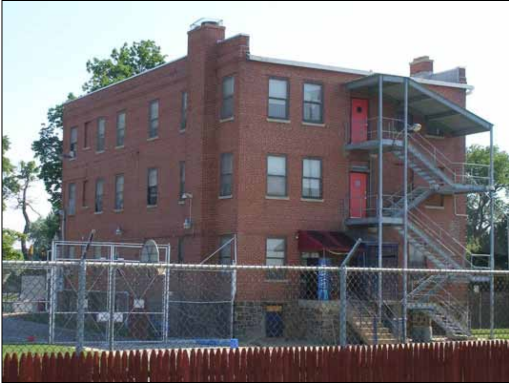
View of the south and west elevations, looking northeast.
