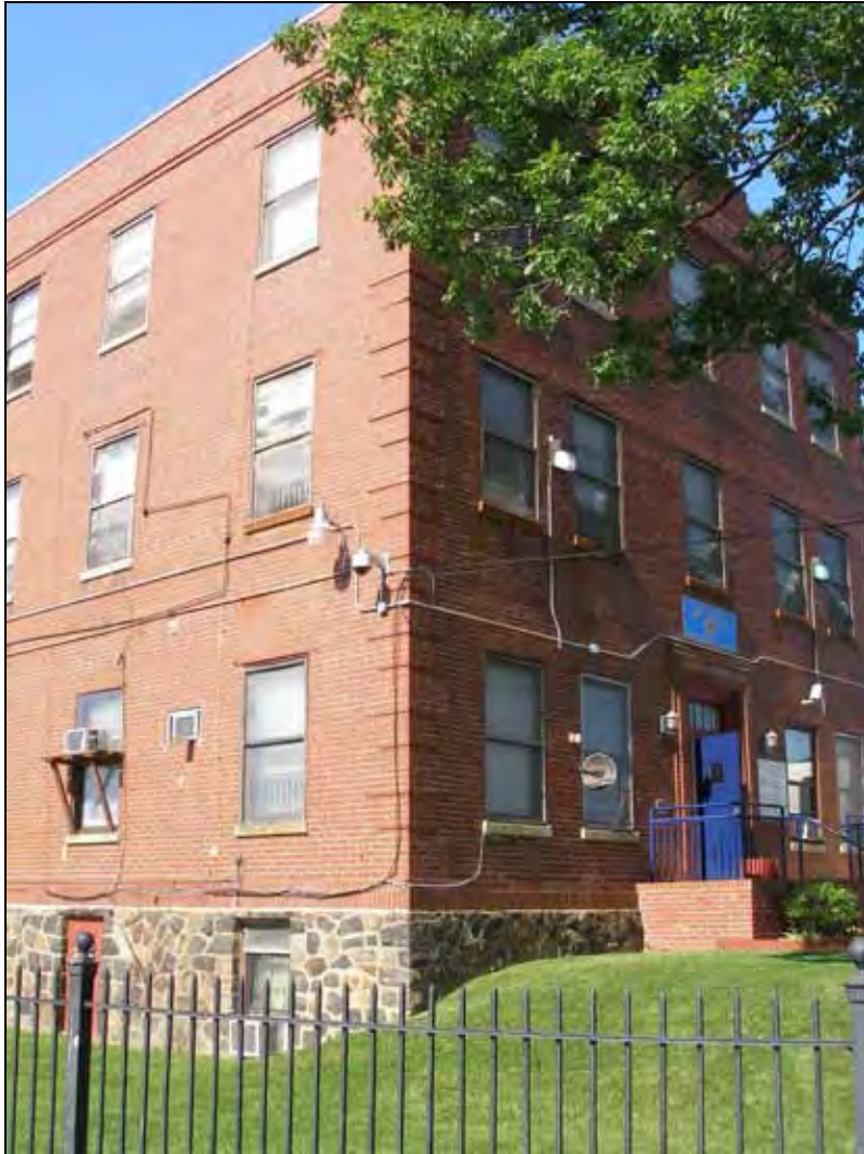
View of the northeast corner of the New Castle County Workhouse – Women's Ward (N-13,728) looking southwest.
