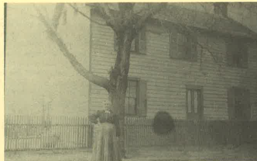
At left: A turn-of-the century photo of the Burge house on South Street. Mrs. Burge is standing out front. 37
