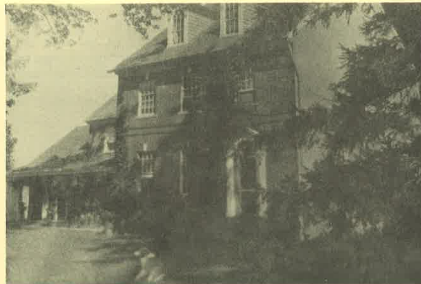
At left: "Brookramble" on The Levels, built by James Crawford in 1805, was the 19th century home of Dr. James V. Crawford and the 20th century home of the George Ginn family. This house is now owned by David and Allison Matsen. 35
