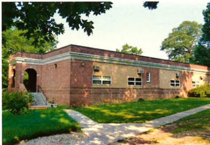
George Wilson Community Center (July 2008)
