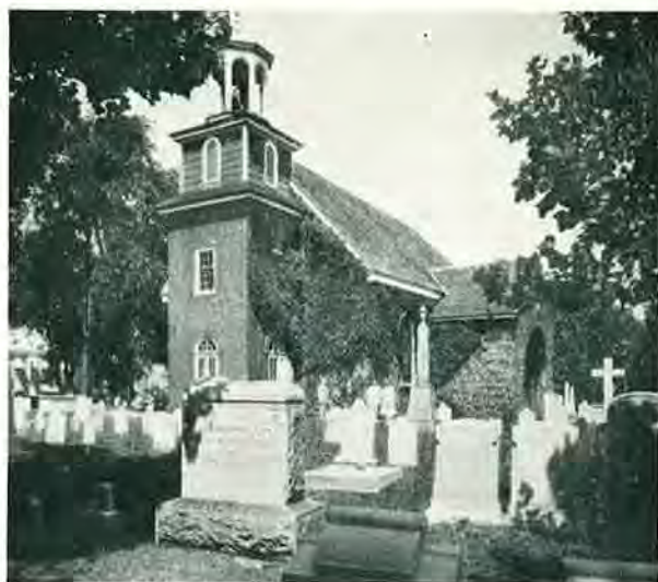
Holy Trinity (Old Swedes) Church, Wilmington, Delaware
