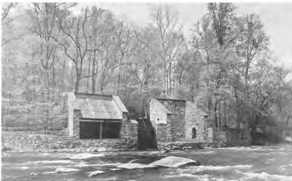
4.—MODEL OF A PAIR OF ROLLING MILLS. This shows how the water which was used to drive the mills mixed the powder. (Below) 5.—THE BIRKENHEAD MILLS BUILT IN 1822-24 AND NOW PARTLY RESTORED. The idea of the three stout stone walls and a light roof and fourth wall was that the wall would blow out over the river if there was an explosion
