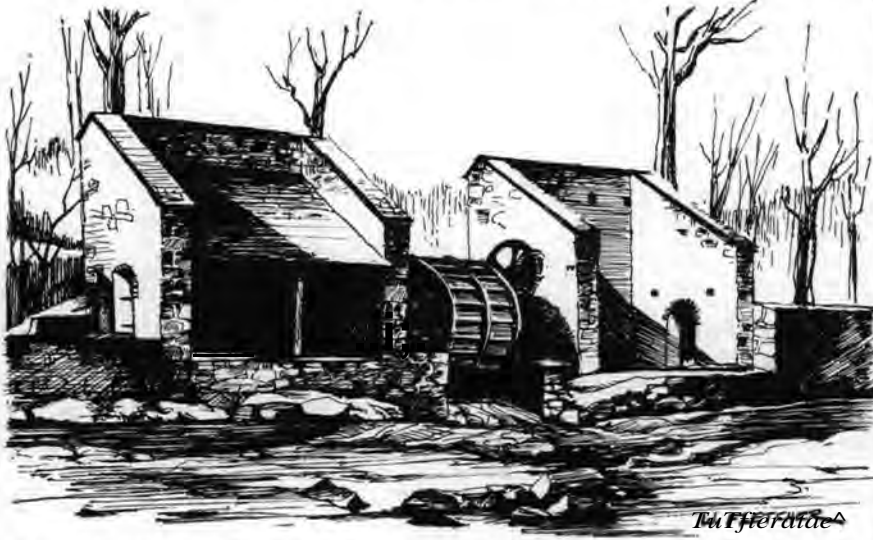
An artist's sketch of the Birkenhead powder mills on the Brandywine as they will appear when the wooden water wheel and roof are reconstructed.
