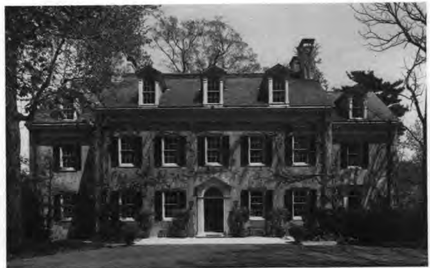
"Eleutherian Mills," built of Brandywine granite and covered with stucco, was designed by Pierre Bauduy, a French refugee from Santa Domingo and early partner of E. I. du Pont.
