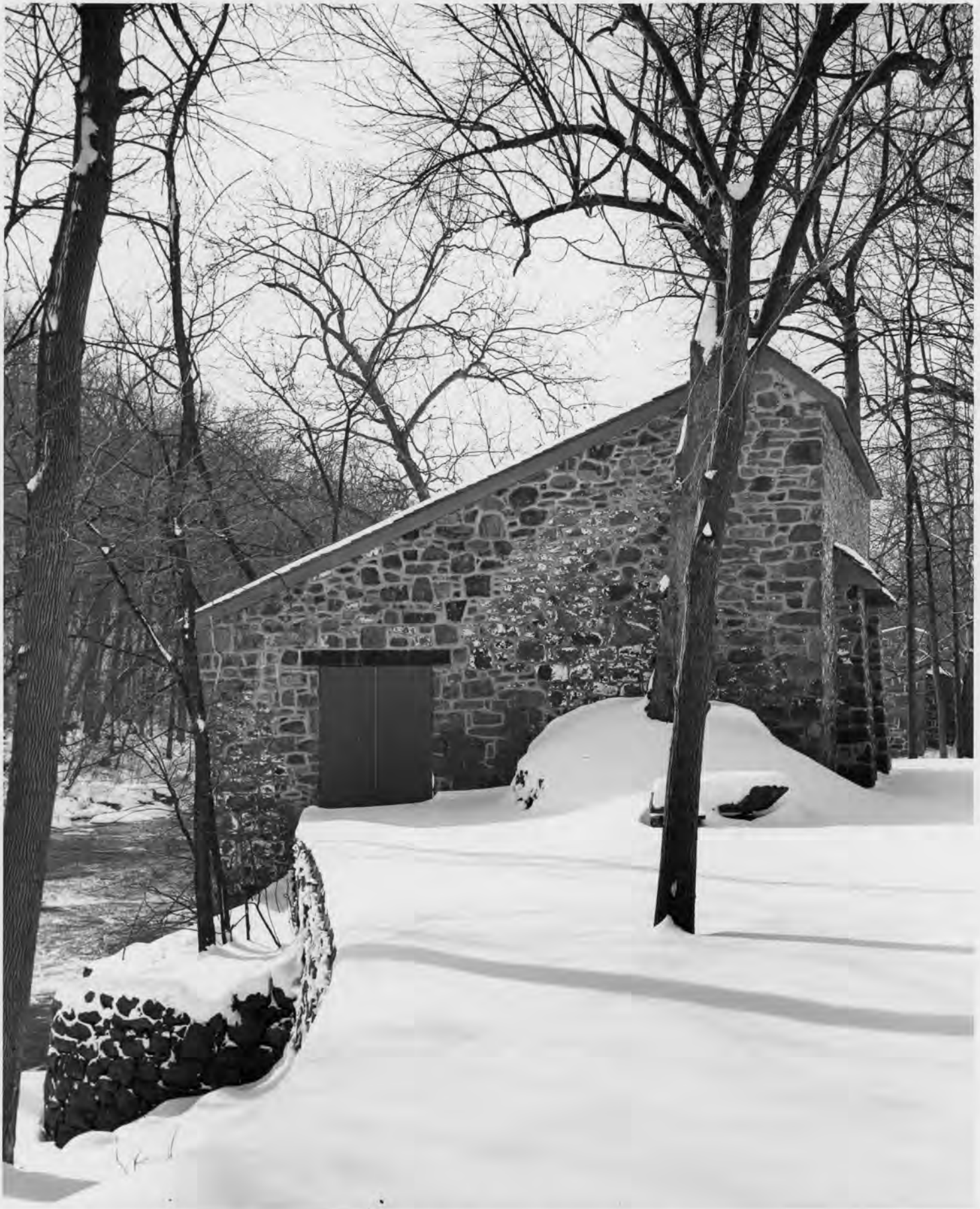
R-13. Glaze Mill - Building shell only. Walls capped in original fashion to prevent deterioration.
