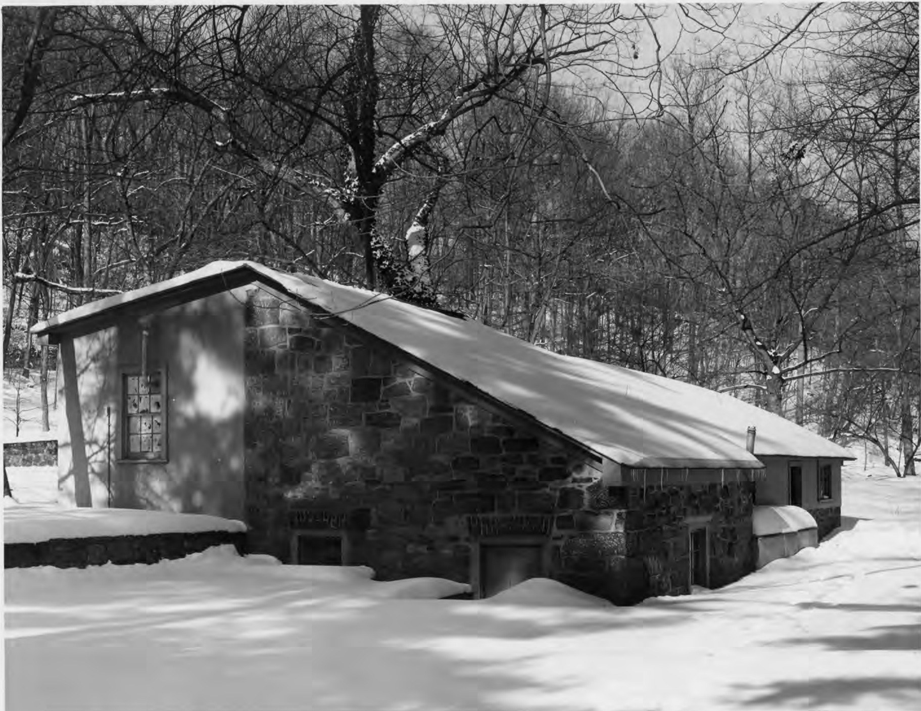
S-22. Sawmill-Pump House - Parts of this building could be the earliest structure standing on the property (reference 1797 map). Wooden superstructure late replacement.
