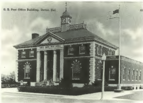
DV12 WESLEY CHURCH EDUCATIONAL CENTER (U.S. POST OFFICE, FEDERAL BUILDING), early view
