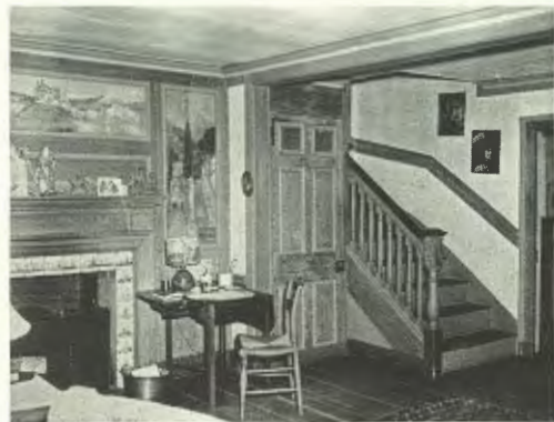
DV13 PARKE-RIDGELY HOUSE, photo c. 1960
