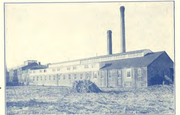
Richardson & Robbins Plant, Dover, Del.
