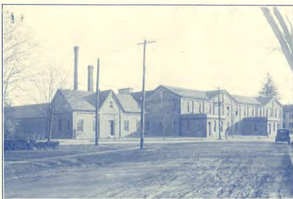
Richardson & Robbins Plant, Dover, Del.
