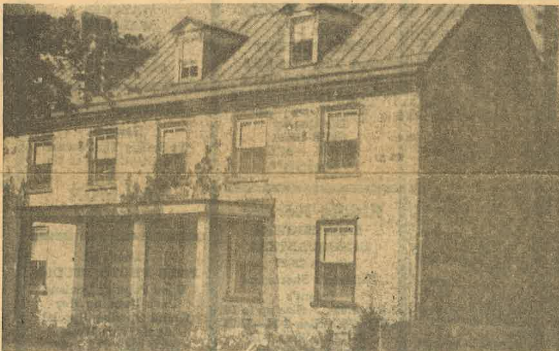
OLD STONE HOUSE, LITTLE CREEK LANDING'S OLDEST STRUCTURE, BUILT BEFORE 1768 FROM BALLAST STONES
