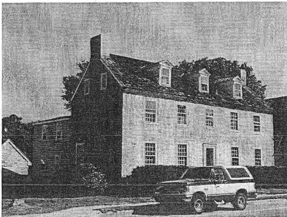
K-0000-2: Perspective of west and north elevations looking southeast showing early nineteenth century stone block, twentieth century shed addition and detached Period I stone outbuilding
