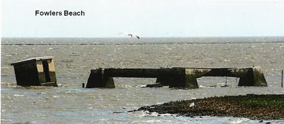
FOWLERS BEACH CABLE HUT AND BASE
