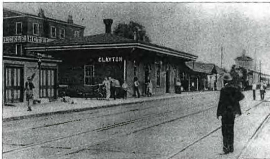
Early postcard view of the Clayton station shows two chimneys on the depot and a platform canopy (to the right), all now gone.
