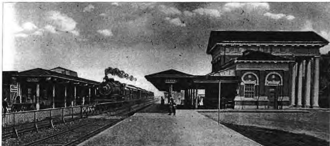
Dover station after its 1911 expansion.
