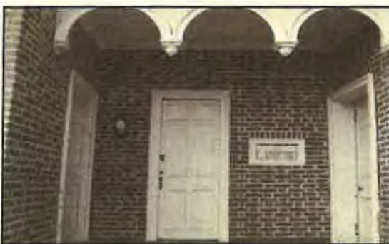
East arcade after completion of brick repointing.
