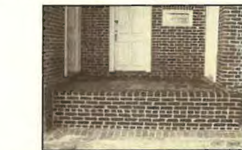
East arcade floor and retaining wall after reconstruction.
