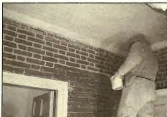
Bill Emory of Roberts Construction repoints the east arcade brick wall.
