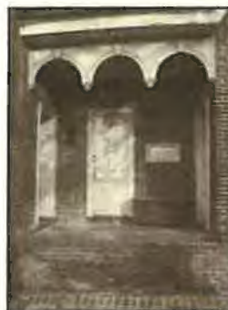
East arcade floor prior to renovation.
