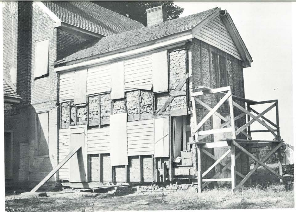
Parson Thorne Mansion undergoing restoration in 1963. Removal of worn siding on this rear wing exposed brick nogging used for insulation.
