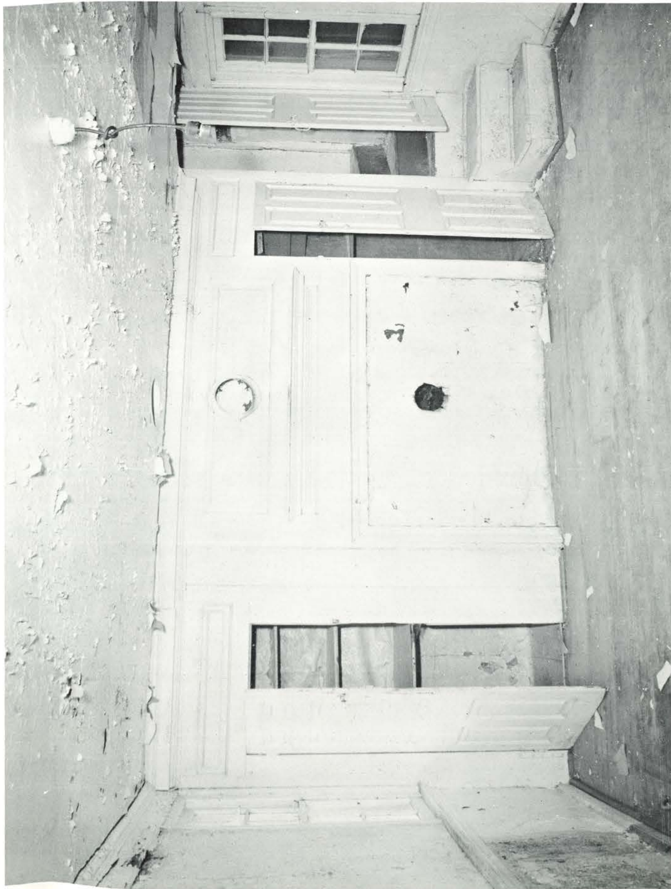
INTERIOR OF REAR WING
