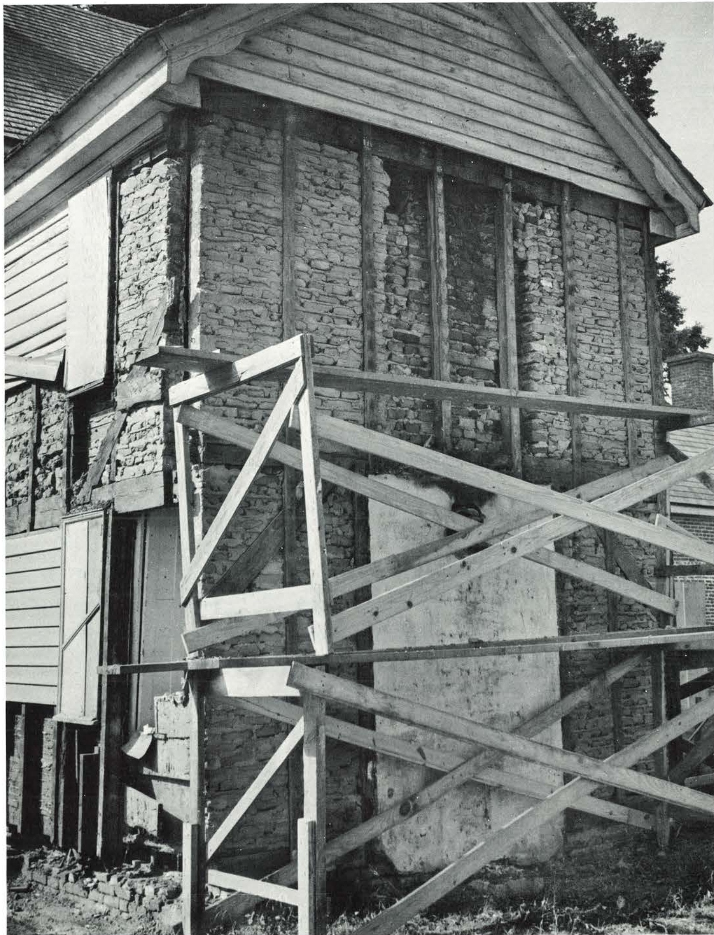
REAR WING UNDER CONSTRUCTION SHOWING NOGGING BETWEEN STUDS
