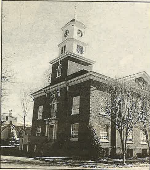
THE KENT COUNTY COURT HOUSE was built in 1874 as a three-story Victorian building and renovated to its present two-story Georgian appearance in 1918. During the renovation, new dials were installed in the new clock tower, but the original clock works remain in place. Photo by Joanna Wilson.
