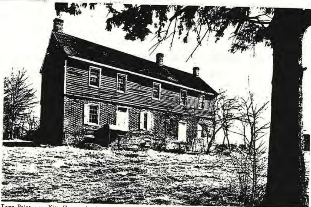
Town Point, near Kitts Hummock, circa 1675. The brickwork is admirable and intact. Note the stepped water-table. The frame upper storey is an early nineteenth century defacement.
