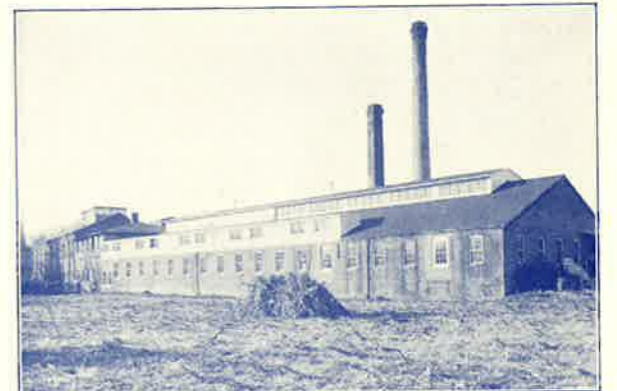
Richardson & Robbins Plant, Dover, Del.
