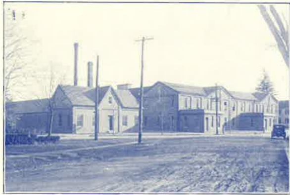
Richardson & Robbins Plant, Dover, Del.
