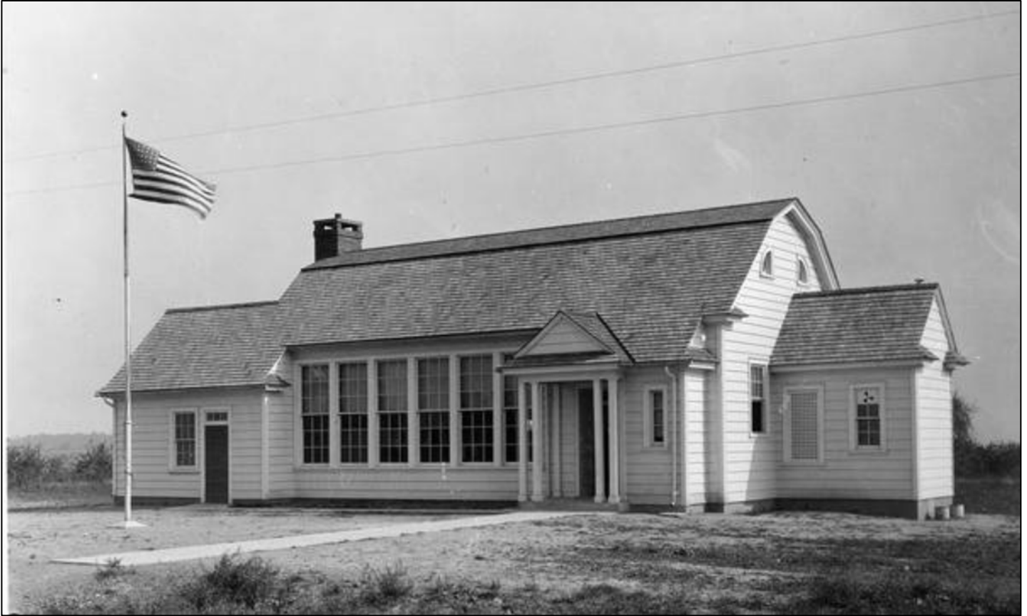
Figure 7. Public School No. 111-C in Christiana (New Castle County), among the first three minority DuPont schools to be constructed and of an experimental model form, c. 1920 (Hagley Digital Archives, Delaware School Auxiliary Association photographs)
