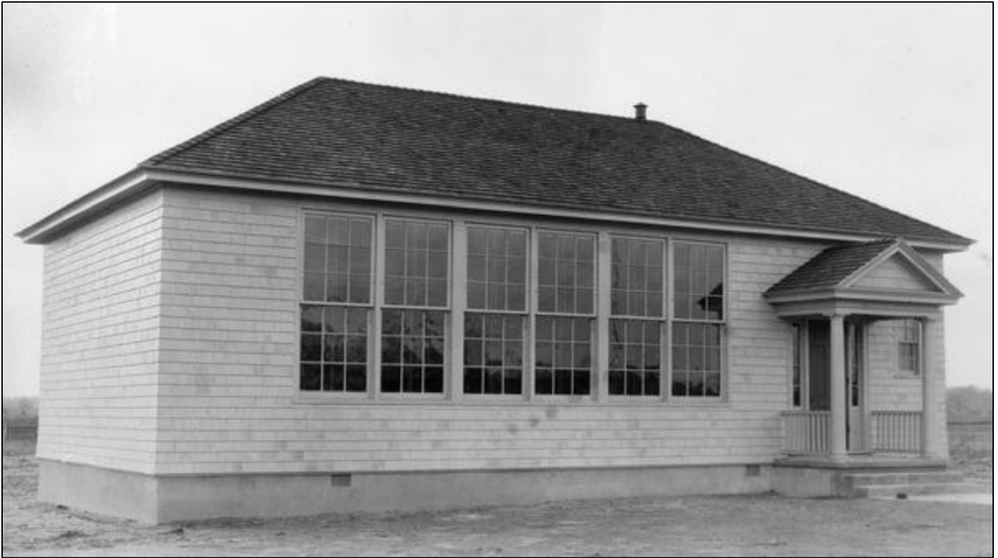
Figure 12. Green Spring School 128-C (New Castle County), showing bank of large classroom windows running to the cornice with five thin mullions separating each window, c. 1922 (Hagley Digital Archives, Delaware School Auxiliary Association photographs)
