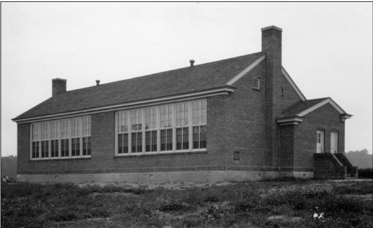
Figure 11. Williamsville-Bethesda School 113/114-C (New Castle County), a two-room plan exhibiting banks of classroom windows to provide appropriate lighting, c. 1927 (Hagley Digital Archives, Delaware School Auxiliary Association photographs)
