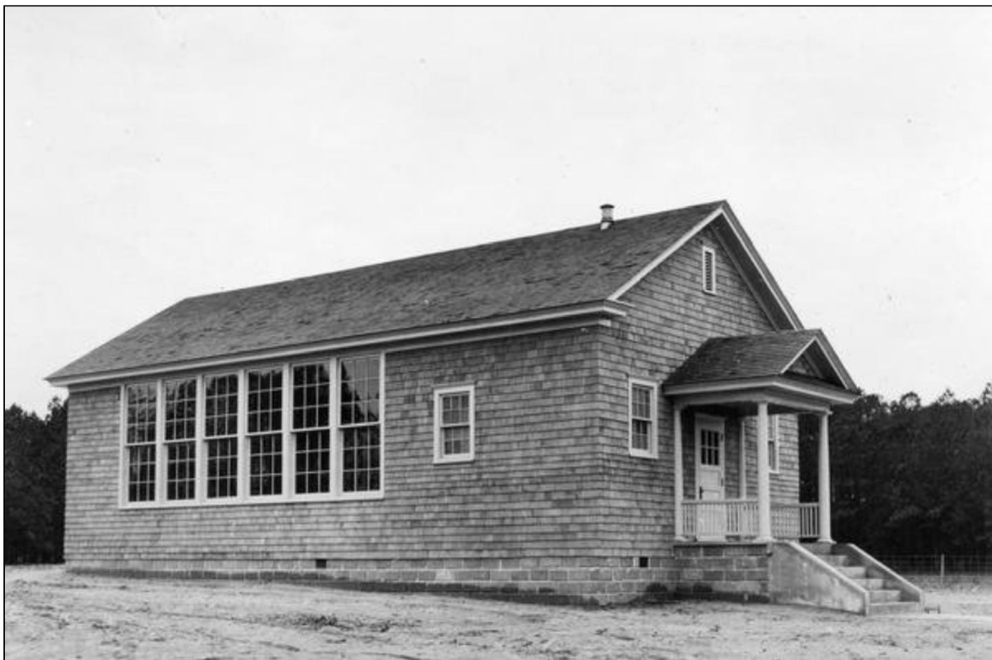
Figure 10. Friendship School 202-C (Sussex County), exhibiting the standard one-room/front-gable design utilized for many of the minority DuPont schools, c. 1922 (Hagley Digital Archives, Delaware School Auxiliary Association photographs)
