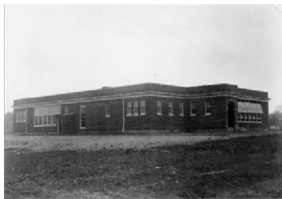
Smyrna Colored School (1921) - This one-story brick school building featured covered arched side entrances and five classrooms. Each classroom had a large bank of six windows. The location was in an expanding community area for African Americans in Smyrna, Delaware. Construction started on January 21, 1921, and was completed on October 1, 1921. (Courtesy of Hagley Digital Museum)
