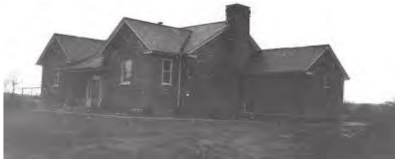
Hockessin Colored School #107C was a one-room, one and a half story brick building with an entrance hallway, a coatroom, and a room for the stove that heated the building. (Courtesy of the Delaware Public Archives)
