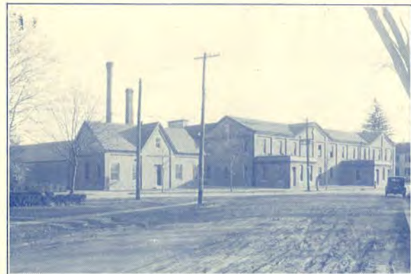
Richardson & Robbins Plant, Dover, Del.
