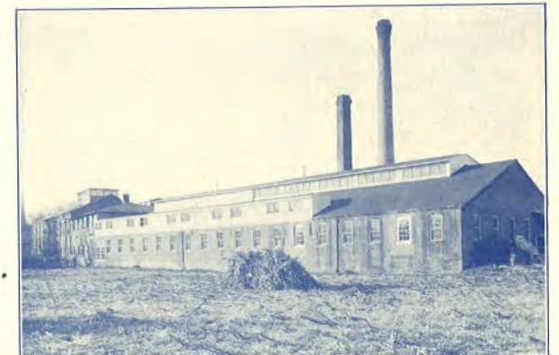
Richardson & Robbins Plant, Dover, Del.
