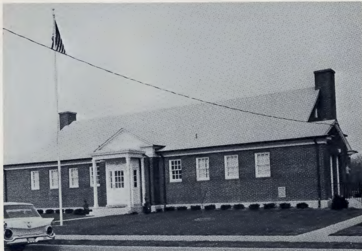
THE NEW ADMINISTRATIVE OFFICES OF THE CAESAR RODNEY SPECIAL SCHOOL DISTRICT, CAMDEN-WYOMING, DELAWARE.
