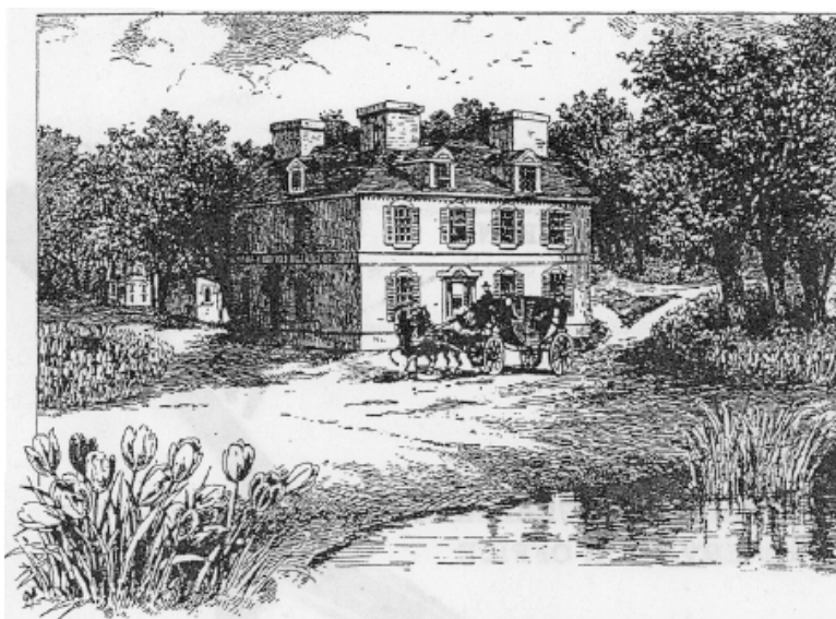
READ MANSION, ON DELAWARE BAY, NEW CASTLE, DEL., IN COLONIAL DAYS
