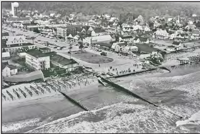
Above: Rehoboth Beach Boardwalk damage 1962 Resource ID: 1325-003-036_00755n
