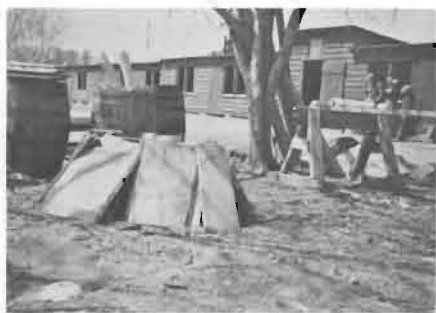
YELLOW PINE SLABS READY TO BE SPLIT INTO FOUR INCH WIDTHS AND SOAKED IN THE BARRELS AT THE LEFT. AFTERWARDS THEY WILL BE SHAVED DOWN INTO SPLINTS TO BE WOVEN INTO UPRIGHTS AND FILLING OF BASKET-WORK EEL POTS.
