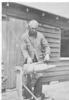
ELWOOD WRIGHT, NOW DECEASED, PERFORMING FIRST STAGE OF YELLOW PINE SPLIT EEL POT ON REVOLVING MOLD.
